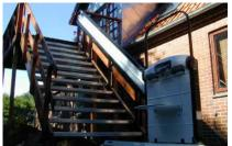
Where space is limited, a wheelchair suitable platform stair lift provides disabled access up to 250kg in a compact way. LEARN MORE
