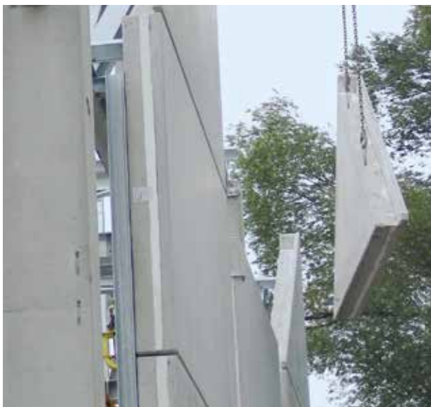
Sandwich wall with Schöck Thermoanker
