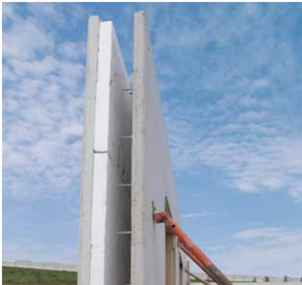
Twin wall with Schöck Thermoanker
