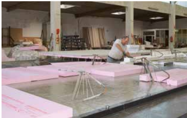
1. Cover the freshly cast concrete outer leaf with thermal insulation
