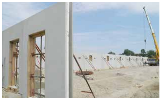
4. Erect wall construction on-site
