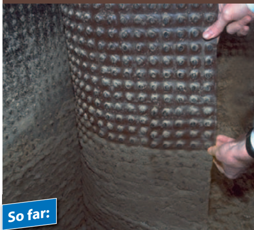
The dimples of many dimpled sheets press against the bitumen coating of cellar walls – a severe stress on the waterproofing.
