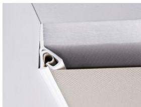
Clipso ceiling installation with PCW profile.
