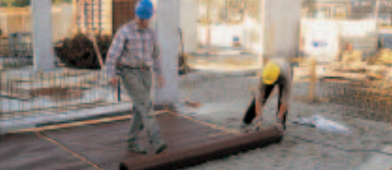
Sheets can be rolled out easily and quickly.
