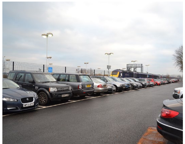
Installed beneath the car parks, ACO StormBrixx provides a sustainable surface water management system.
