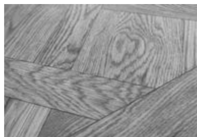
Versailles wood structure *
