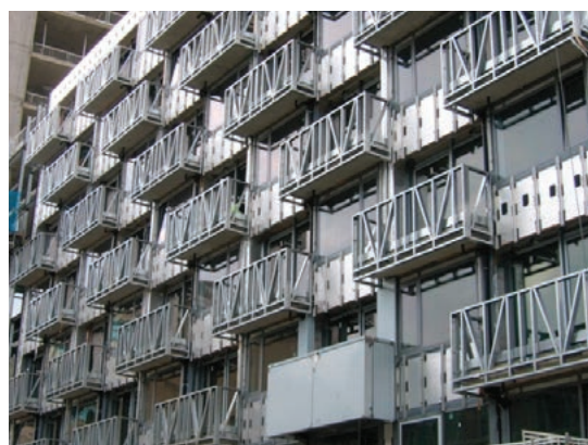
Figure 10.3 Light steel external walls with integrated balconies
