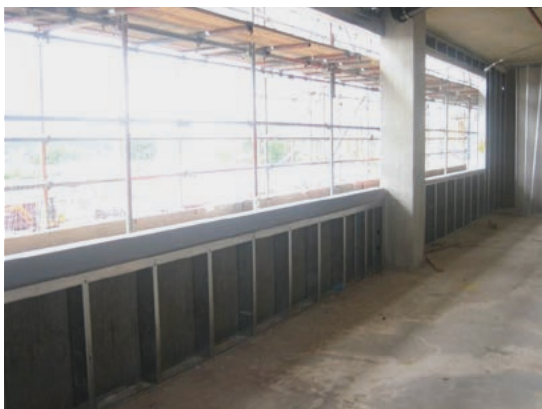
Figure 10.2 Large ribbon window in infill panel
