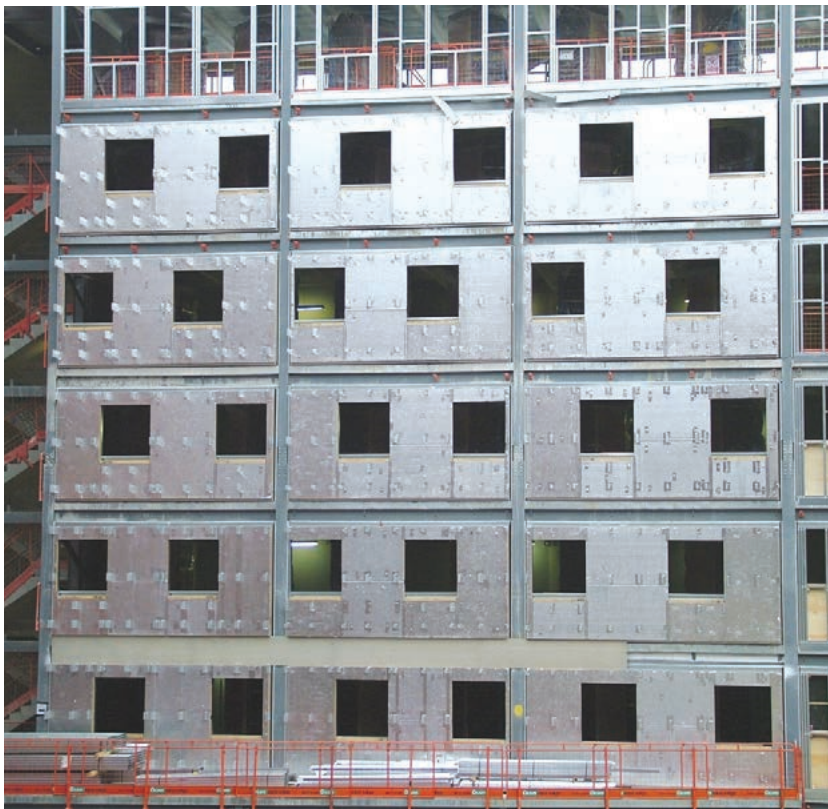
Figure 1.3 Typical prefabricated panelised external infill wall system
