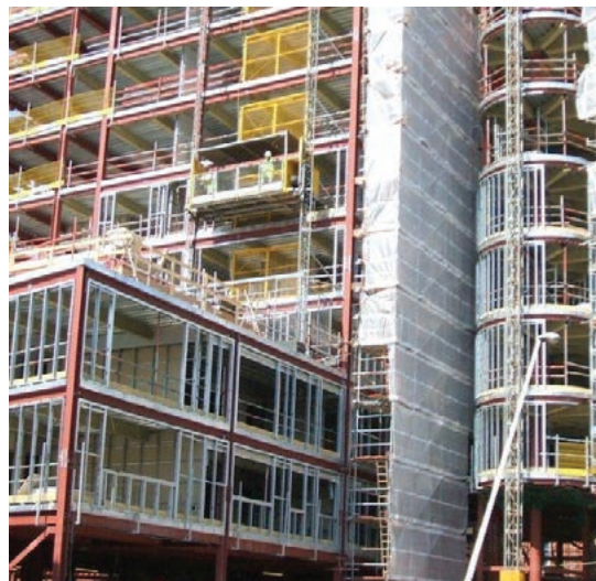
Figure 10.1 Curved infill walling - during and after construction
