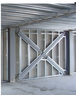
Figure 3.6 Infill walling around primary bracing
