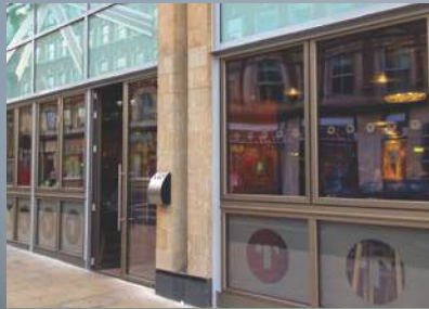
Finished in anodised Bronze with metallic RAL beading with satin nickel hardware.
