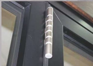
High security hinges, non face fixed.
