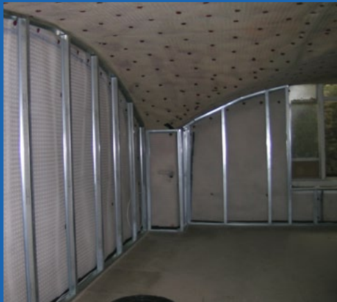
Newton 508 has been applied to the walls of this domestic basement
