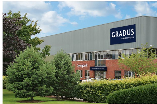
Gradus Springbank - Manufacturing plant for Accessories Macclesfield Cheshire UK
