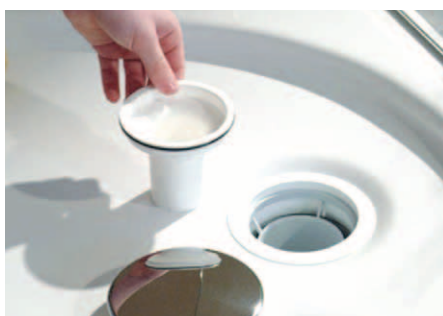
Remove trap insert
