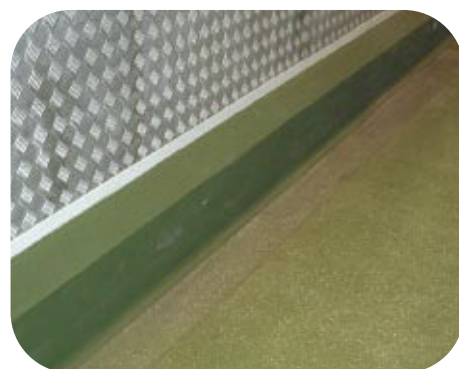
Rendered Concrete Kerb
