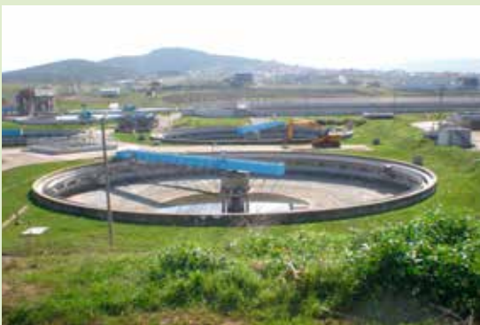
Sewage treatment plant, Istanbul, Turkey
