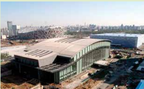
Olympic hall, Beijing, China
