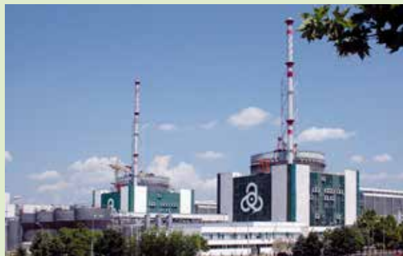
Nuclear power station, Sofia, Bulgaria
