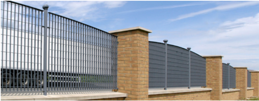
Roma-3 Bespoke Perimeter Fencing Manor Business Park, Banbury
