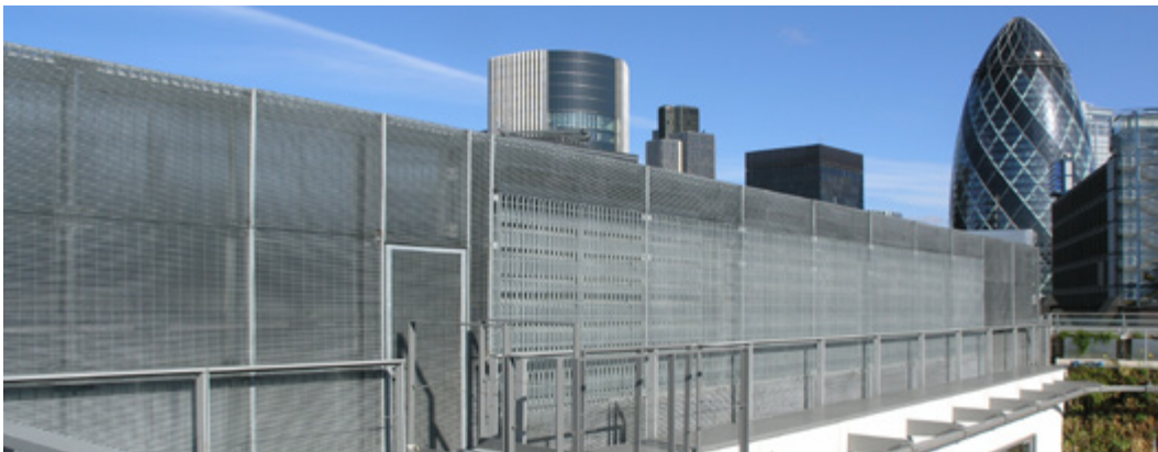
Micro-15 & Stereo-4 Roof-top Plant Housing Hilton Hotel, Tower Hill
