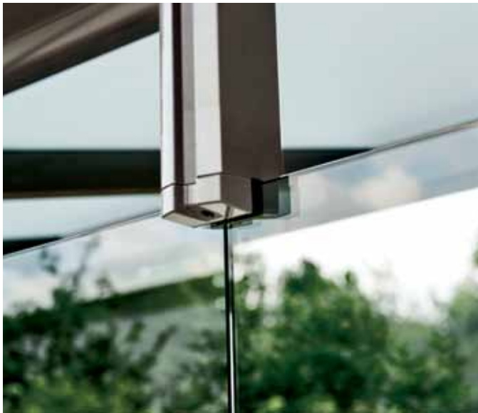
Connect glass panels offer: safety, protection from wind and rain, unimpeded egress. Panels may be patterned to signal their presence and avoid walk-in collisions.
