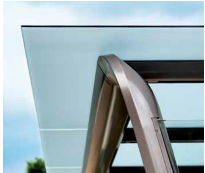
Smoked grey roof panels made of tempered glass with mylar film laminated between sheets, block 80% of UV rays.
