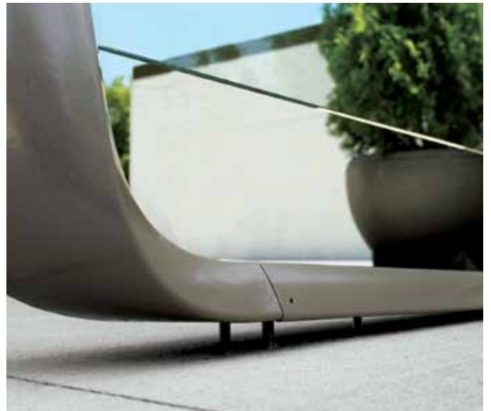
Leveling anchor rods and bolts are concealed in base plates.
