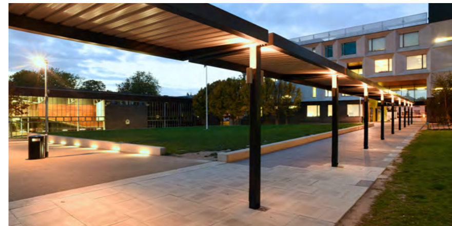
Burntwood Cantilever Walkway BXDB/BURNT-WALK
