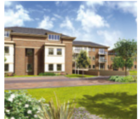
Newton 403 HydroBond was used to waterproof this extensive housing development in Surrey
