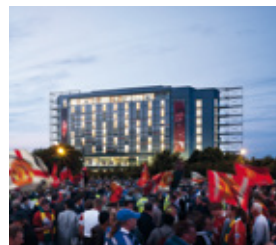
Multiple Newton products were installed in combination to protect the Hotel Football against water ingress
