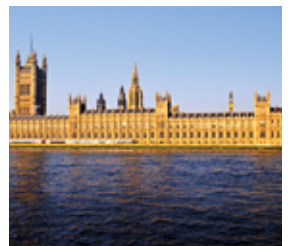
Newton System 500 and Newton 403 HydroBond were applied to the Houses of Parliament, London
