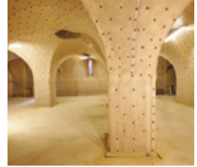
Newton System 500 has been installed in the Grade I Listed Royal Courts of Justice, London
