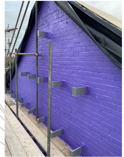
5.1.4 Retrofit- Passive Purple installed insulation
