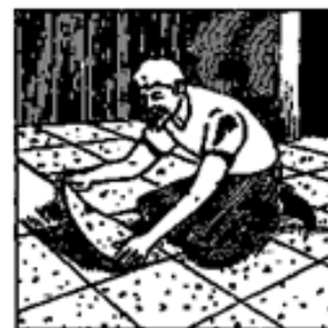
Glue the tiles down
