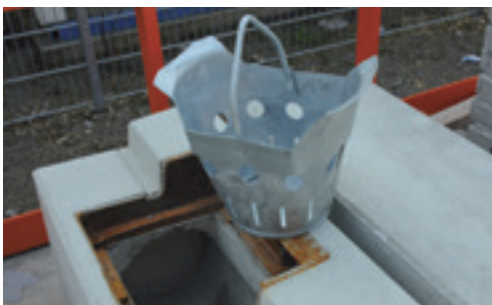
Installed sump unit
