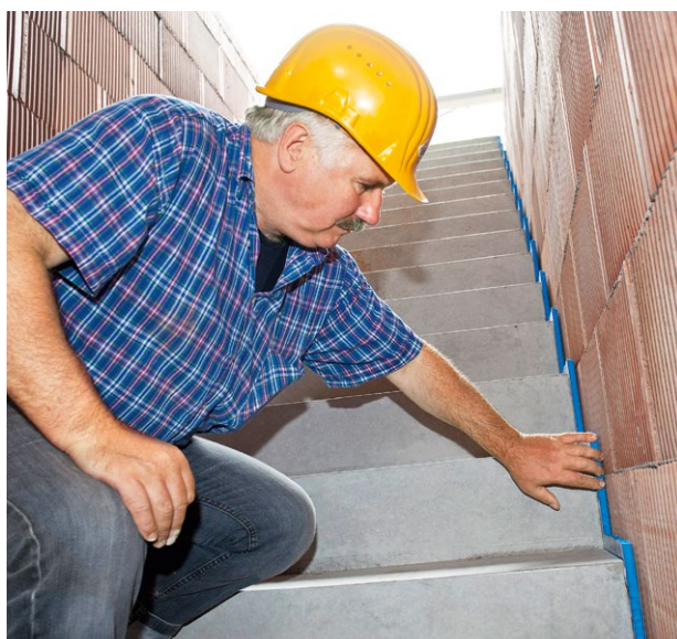
The Schöck Tronsole® types form a blue line in the system. This line denotes the technical approval of the sound bridge-free connection.
