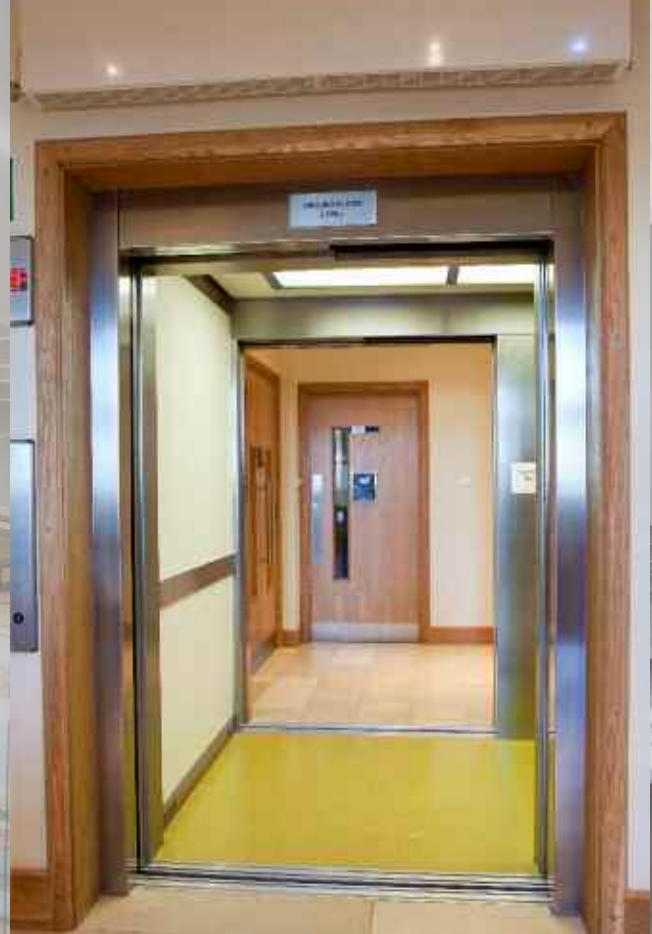
This hospice bed lift with through-car arrangement replaced a conventional single entry lift
