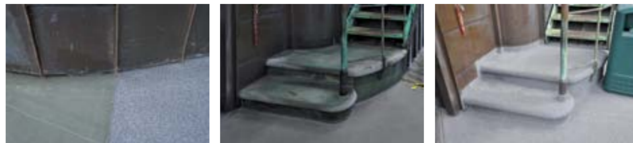
The observation deck of the Hamburg Michel was effectively waterproofed using KEMPEROL® and given hard-wearing-coating using KEMPERDUR®. Round shapes and many complex details-ideal for the application of liquid applied waterproofing
