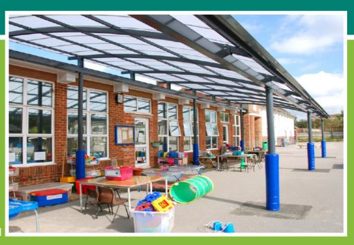
The 16mm triple clip polycarbonate system is used to create a hard wearing roof covering for our canopies.
