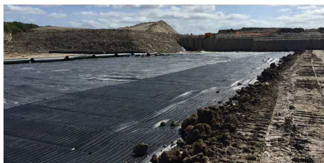
ParaLink® used over mine workings in the South West
