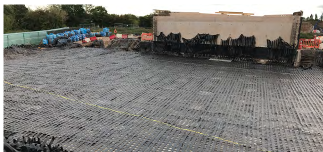
ParaLink® used over piles at Colley Lane, Somerset
