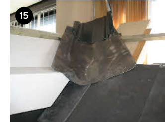
15 Nail on GRP valley tray or form lead valley ensuring a minimum of 150mm cover to lead saddle
