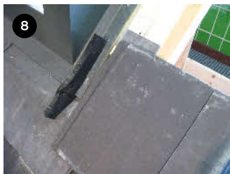
8 Dormer is supplied with 300mm section of self adhesive expanding foam
