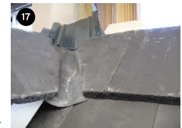
17 Nail on GRP valley tray or form lead valley ensuring a minimum of 150mm cover to lead saddle
