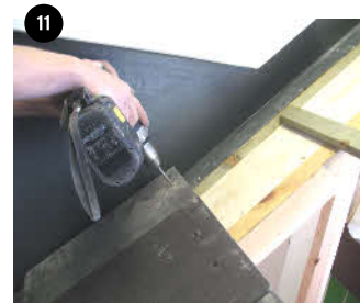
11 Drill and screw all abutment tiles and adjacent tiles
