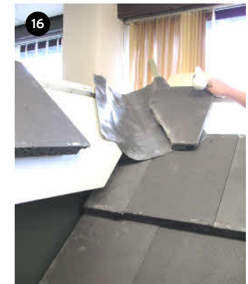
16 Cut valley tiles according. Bed as necessary onto GRP valley tray or on to cloaking piece placed onto lead. Ensure a drainage channel is kept behind mortar bed.
