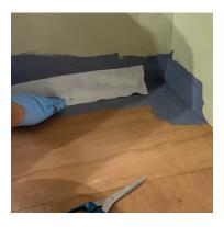
Apply a generous coat of the Compound into the joint area. Then take a pre-cut piece of Super Fleece and push it into the junction – half on the wall, half on the floor – overlapping the corners by about 5cm.
