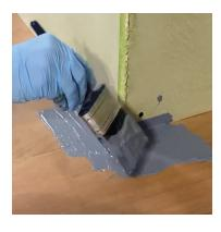
Step 5: External Corners are dealt with in a very similar manner. Start by spreading a generous coating of the BD50 Compound.
