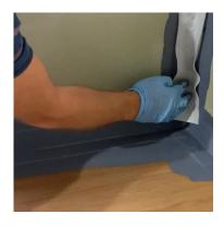
Wall to wall junctions also need to be reinforced and handled in exactly the same manner. Continue until all joints and junctions have been reinforced with the Super Fleece and have been overcoated with the BD50 Compound.
