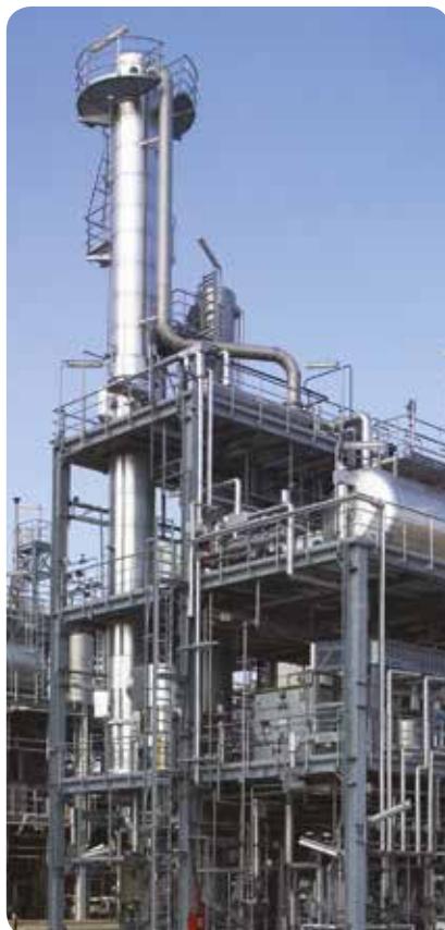
Chemical processing plants
