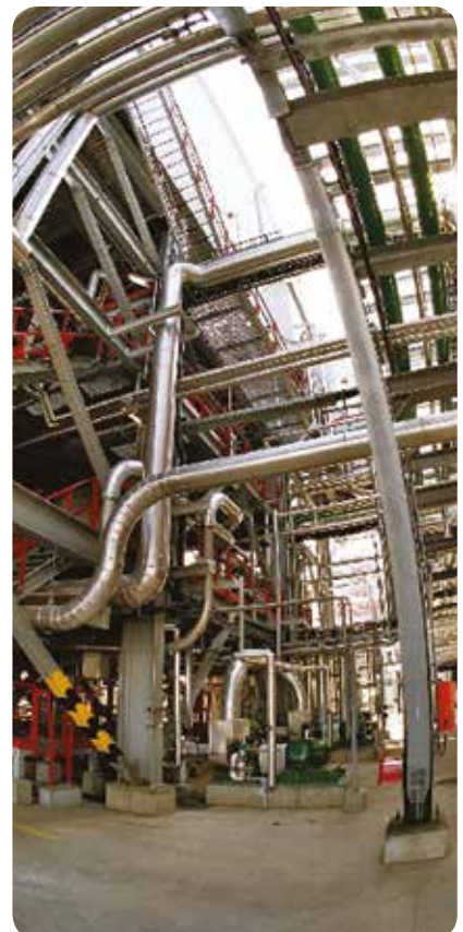
Metal structure coatings
