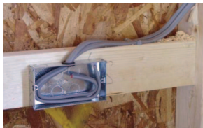
VCL patch behind services in external walls
