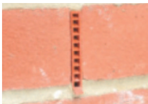
Vents in brickwork above ground level
