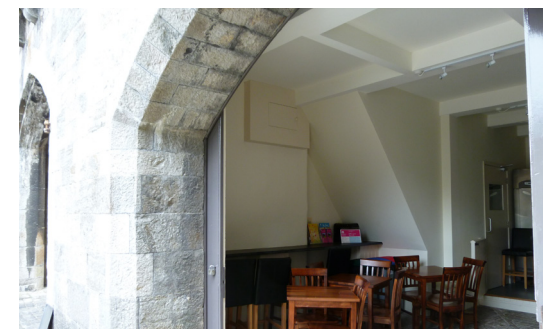
The outbuilding is now free from damp problems and has been converted into a cafe
